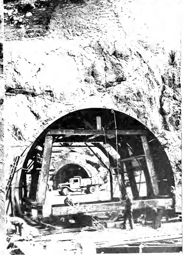
At left, portal of tunnel No. 2 through ridge of Mt. Williamson. This is a 14 x 14 foot pilot bore. At right, top, equipment mucking at main heading of tunnel No. 1, showing protective shell in use. Below, Construction yard between tunnels. Building concrete tunnel lining form. In the background may be seen the portal of tunnel No. 1.
